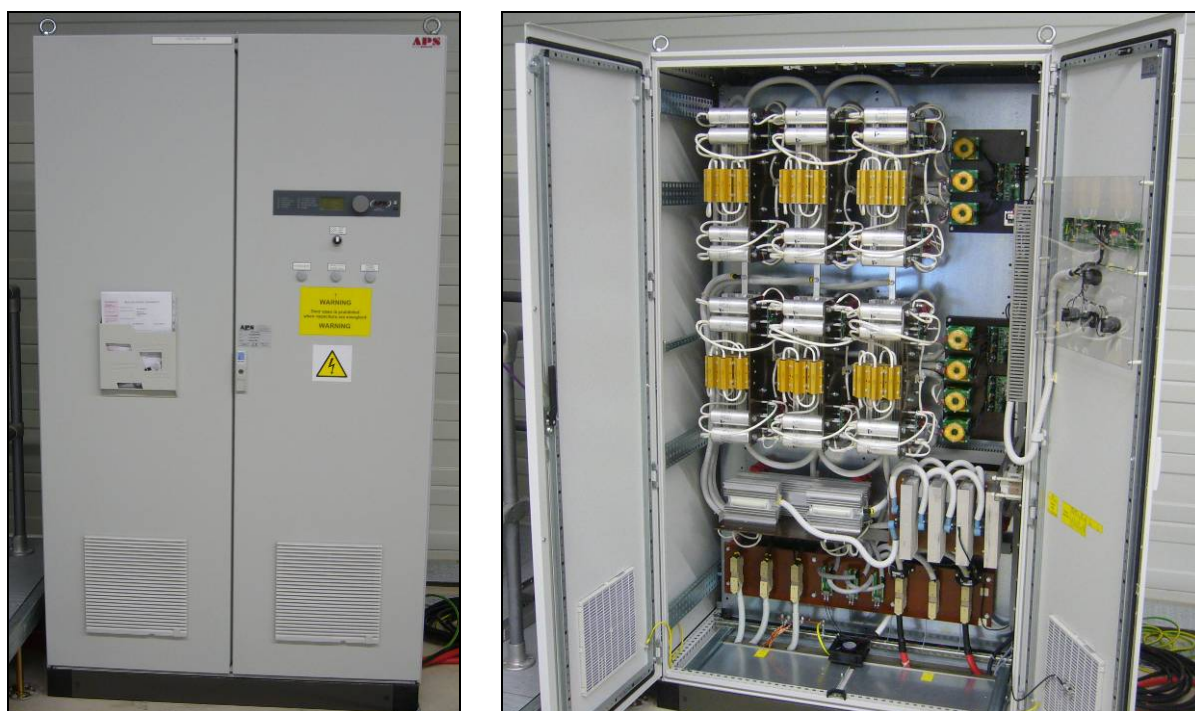
Fig. 3: Delivered low-power medium-voltage dc supply
